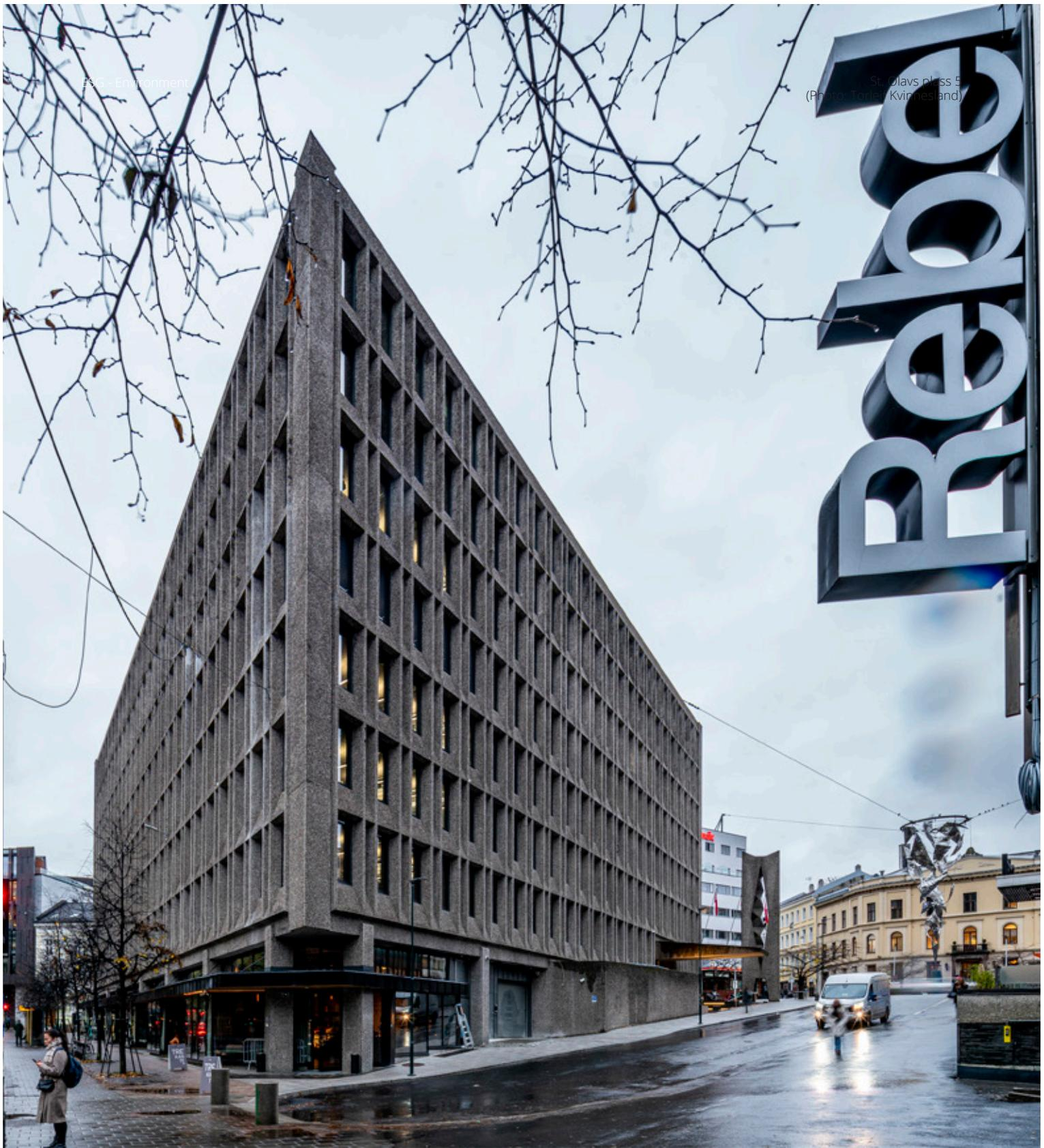
St. Olavs plass 5 was designed by the well-known architect Erling Viksjø and originally constructed in 1967. The building is located in the Oslo city centre and was renovated in 2022. The renovation works included additional insulation, new energy-efficient technical installations and new windows. Even though the building is listed and thus limited the alternatives for energy saving solutions, energy use was improved by more than 50
