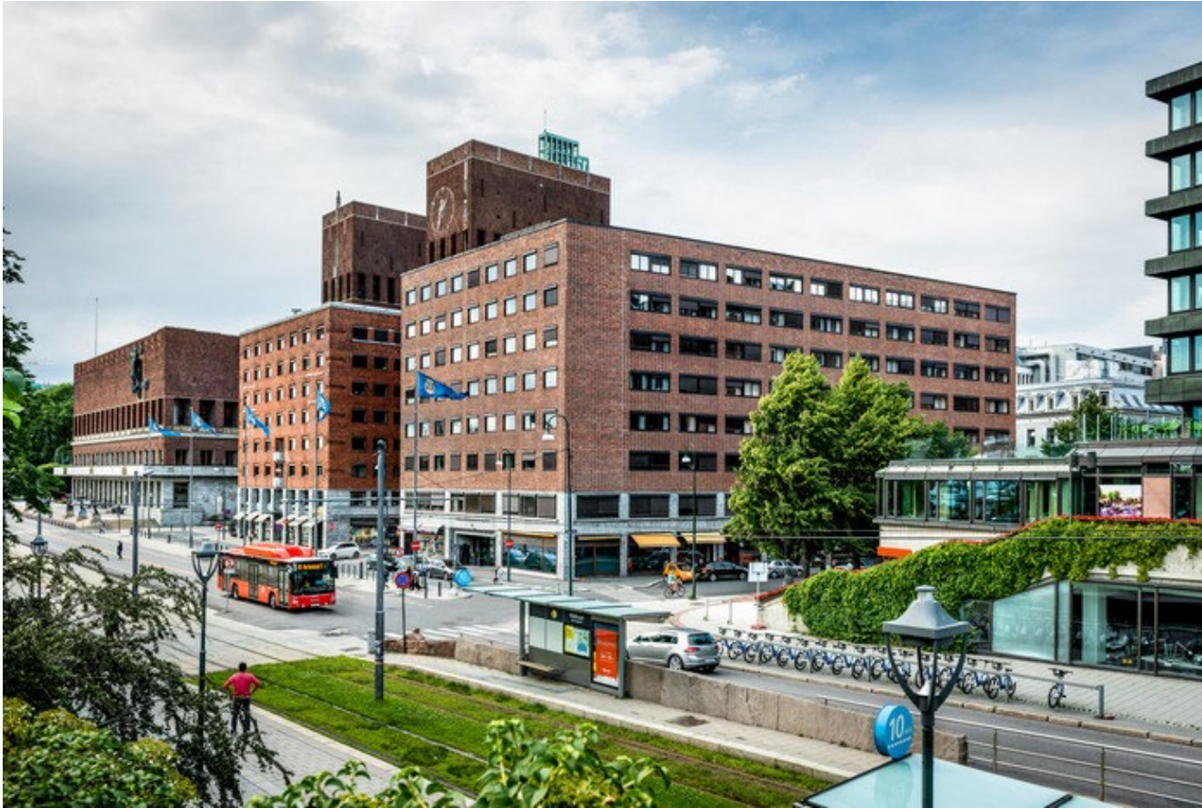
Tordenskiolds gate 12, Oslo
