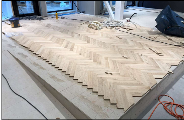
Stavparkett under legging. Foto: Rune Andersen
