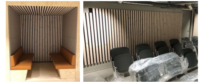
Completed booths and cladding made of used slats on the back wall of the cinema room. Photo: Rune Andersen
