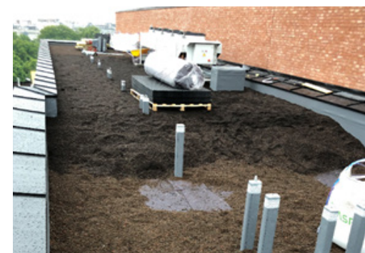
Recycled soil placed on the roof. Photo: Rune Andersen
