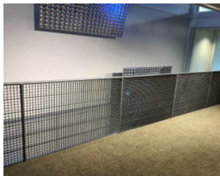
4: Completed railings against the light shaft. Photo: Rune Andersen
