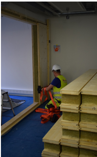
Assembly of the Tewo walls. Photo: Anne S Nordby and Catriona Shine
