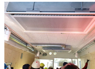
Complete installed beams in the test room of KA13. Photo: Christoffer Siopan Engstrø
