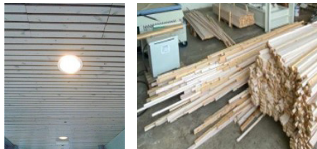
Wooden slats dismantled from the ceiling in the corridors of Refstad school. Photo: Anne S Nordby Storage and production at LUN. Photo: Lars Ulrich Nielson
