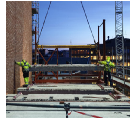
Lifting the hollow core slabs into place. Photo: Mattias Johnsson
